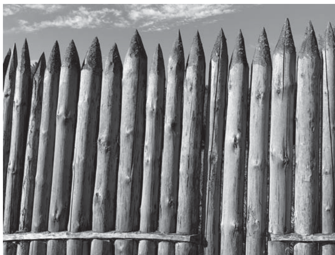
Fig. 5. Restored palisade wall of Fort Umrevinsky.
