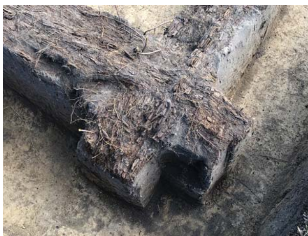
Fig. 7. Logs of a log house joined by the saddle notch (from the northwest). Photo by A.P. Borodovsky.
