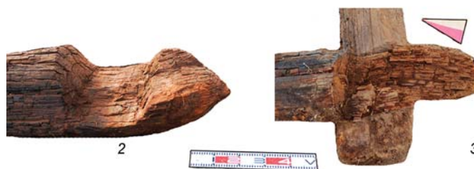
Fig. 6. Visual reconstruction of details of the internal layout (1), design of the end of the log with the saddle notch (2), and saddle-notch joint (3).
