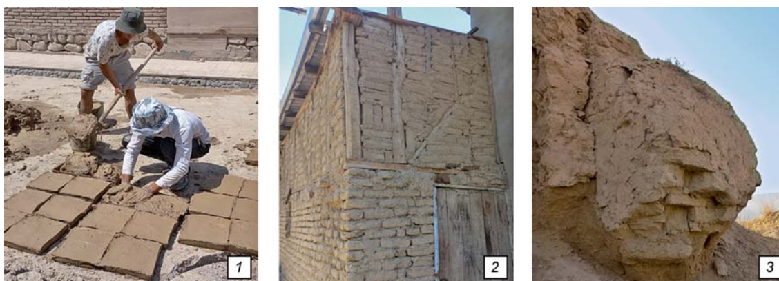
Fig. 7. Construction from adobe bricks. Tajikistan. Photo by N. Petrova. 1 – city of Khujand; 2 – village of Punuk; 3 – fortified settlement of ancient Penjikent.
